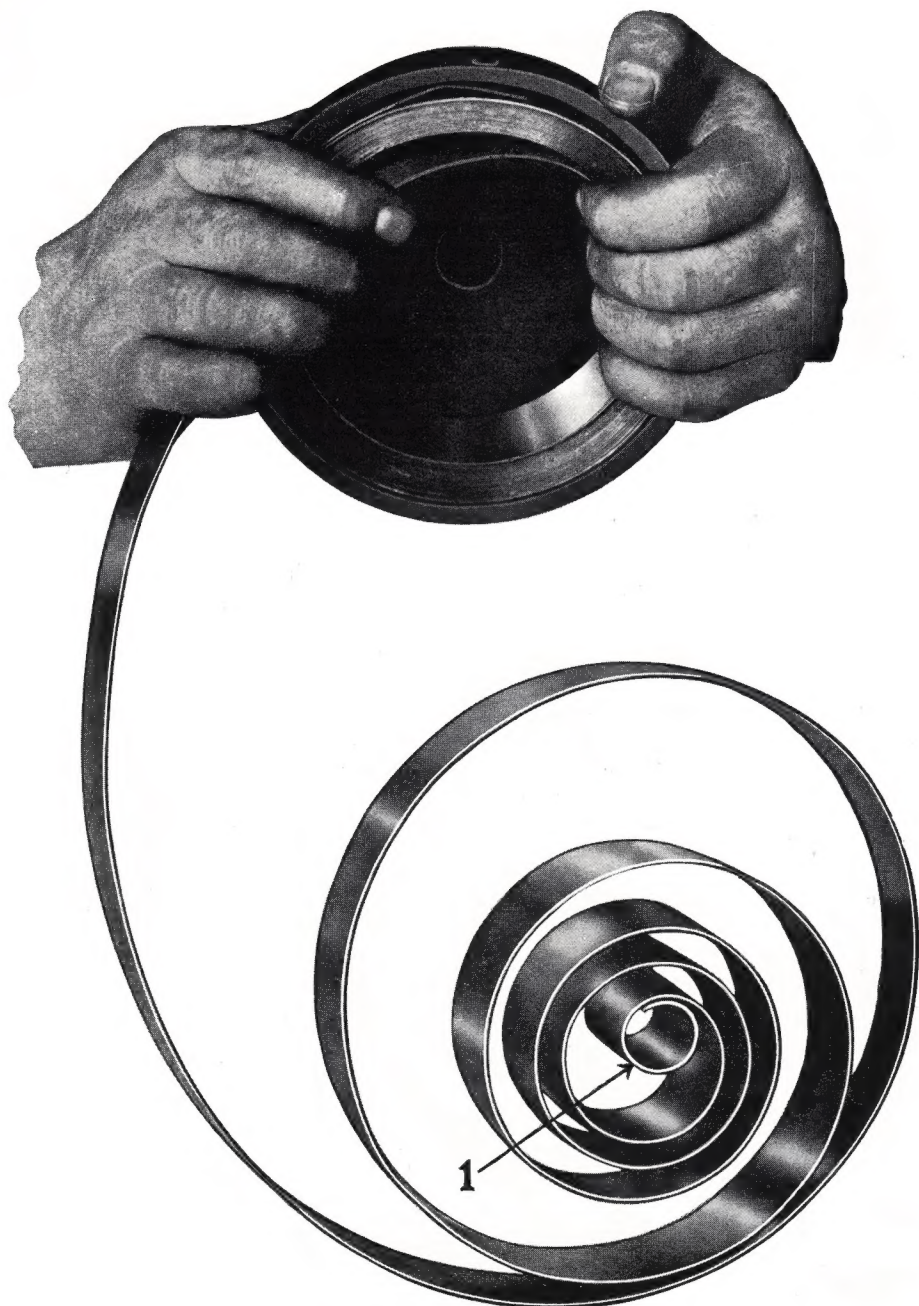
Figure 3—Removing Spring from Case
